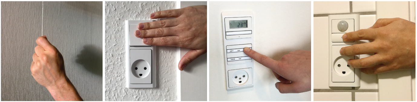
Figure 2. Current ways to interact with light. From left to right: a string-actuated pull switch, a rocker switch, an electronic switch, and an integrated motion detector.
